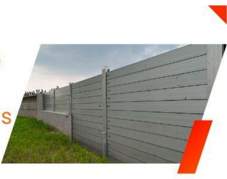
Demountable flood barriers have emerged as a preferred solution for both permanent and temporary flood defense needs. Unlike traditional fixed barriers, these systems can be installed only when required, offering superior flexibility without compromising on strength or performance.
